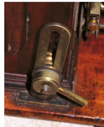
6. Rotary clamp at right front corner of lantern body, guiding it during tilting and securing it in its elevated position
