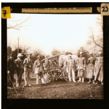
8. Ballard's Fruit Farm employees dressed in old clothes for the task of hot lime washing fruit trees, using an improvised pressure pump on wheels made by adapting a farm cart chassis
