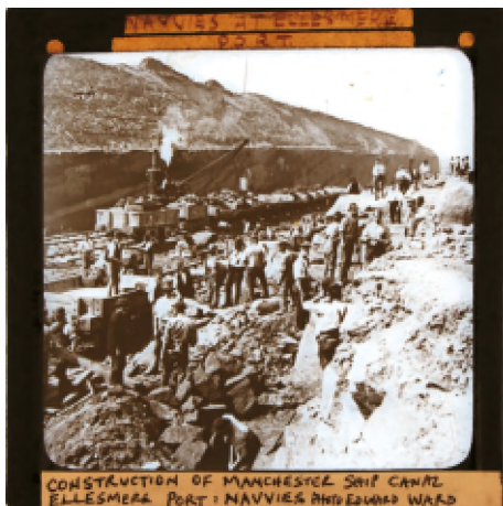
5. Teams of 'navvies' at work clearing spoil by hand during the construction of the Manchester Ship Canal. Photo by Edward Ward of Manchester, late 1880s
